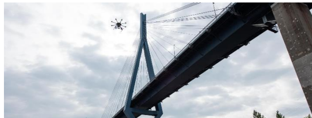
Fig. 10: Drone inspecting an elevated bridge, DLR
