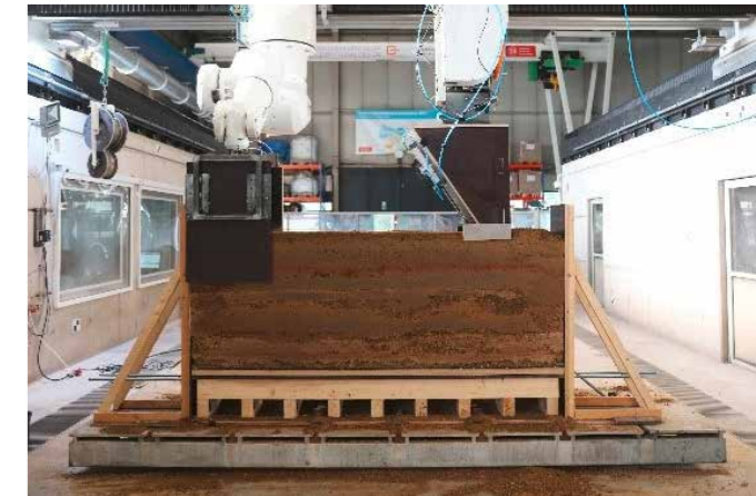
Additive Manufacturing with earthen materials left: Sprayed Earth Additive Manufacturing; right: Robotic Rammed Earth
